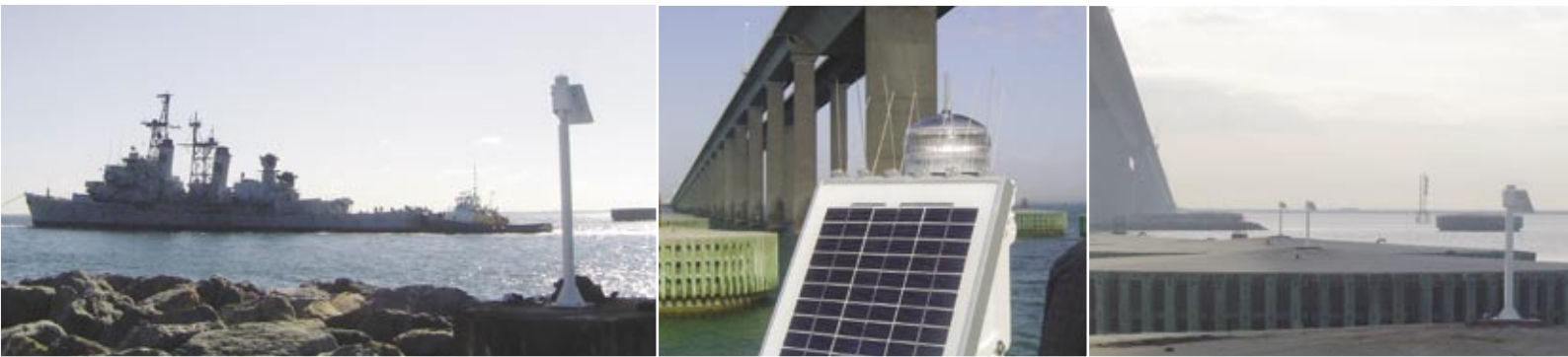
SL23 Bridge Lights, Sunshine Skyway Bridge, Tampa Bay, Florida, USA
